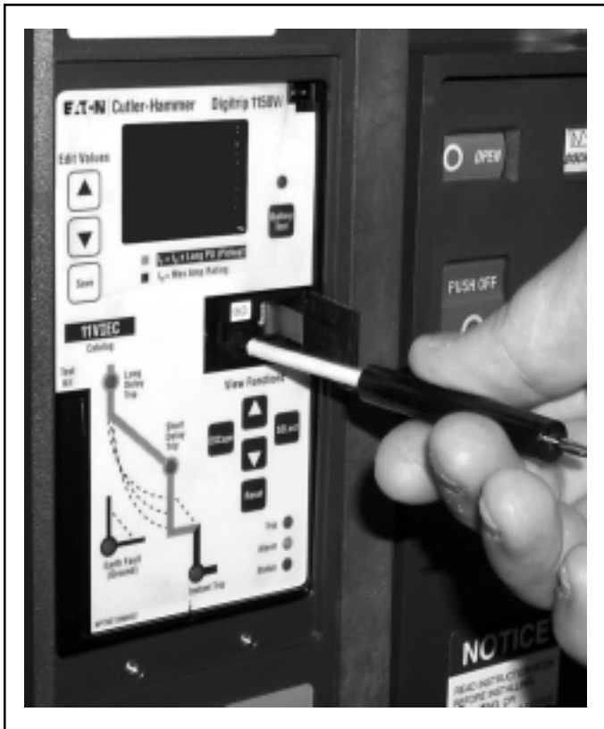
Figure 1.3 Installation of the Rating Plug and Mounting Screw
