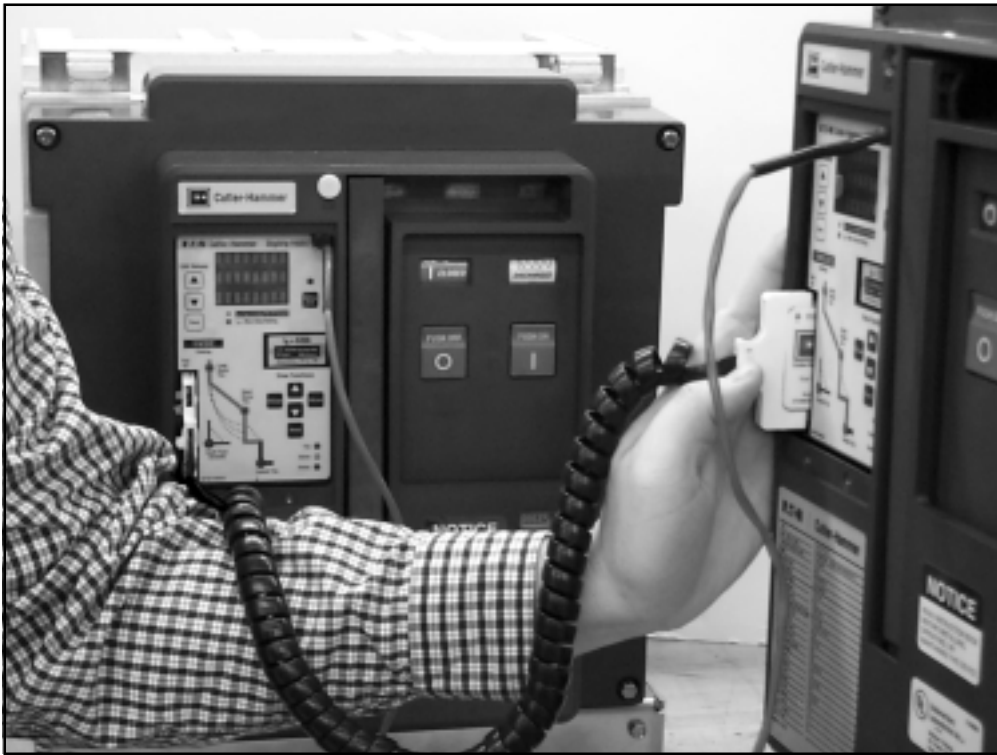
Figure 4.9 TripLink Transfer as shown with Two Type VCP-T Circuit Breakers
