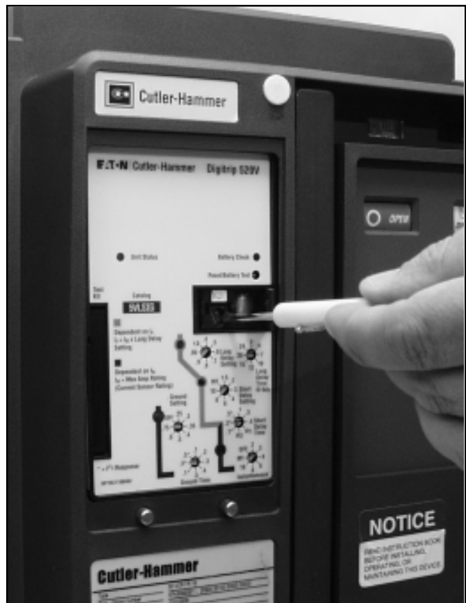
Figure 1.3 Installing the Rating Plug & Mounting Screw
