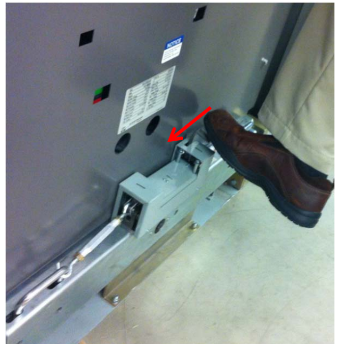
Fig 4-3: STEP – C: Releasing the cradle arms by depressing the “Push Release paddle” towards left.
