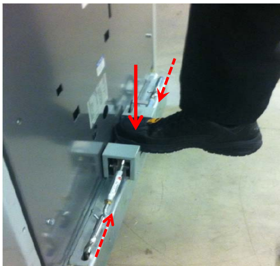
Fig 4-1: STEP – A: Operation of the Cradle Assist Kit
