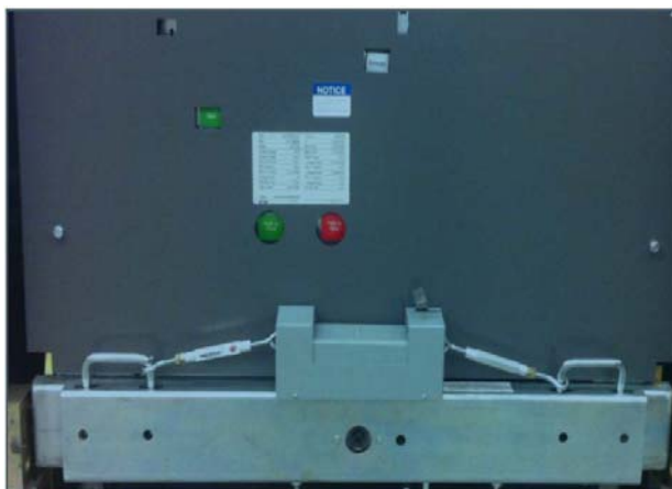
Fig 3-6: Front view of Cradle Assist Kit engaging the VCPW-HD breaker.
