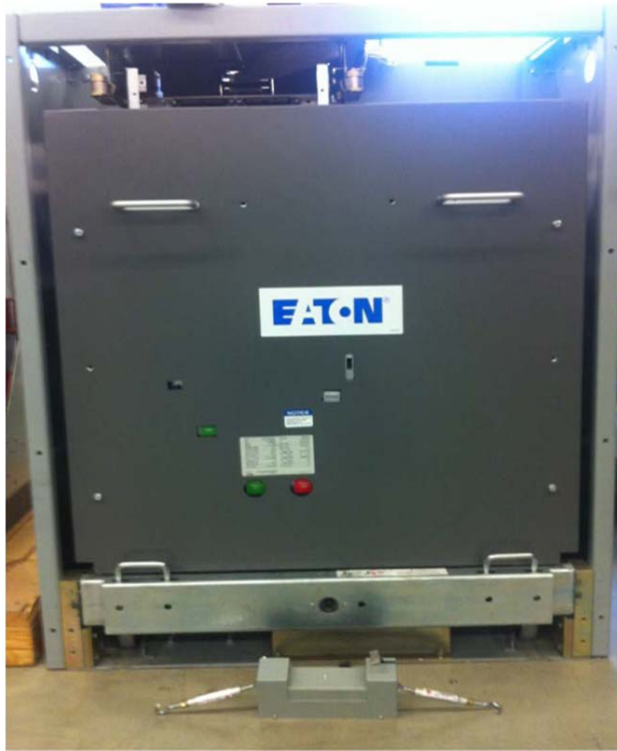
Fig 3-1: Cradle Assist Kit with VCPW-HD breaker with “Pull and Push” type cradle
