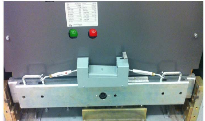
Fig 4-2: STEP – B: Front view of the Cradle Assist Kit pulling the cradle handles and self-locked position.
