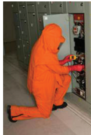
Without arc energy reduction, higher rated and cumbersome PPE as shown, is often required.
