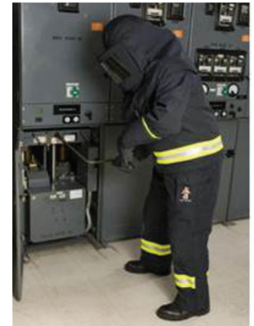
Without arc energy reduction, higher rated and cumbersome PPE as shown, is often required.
