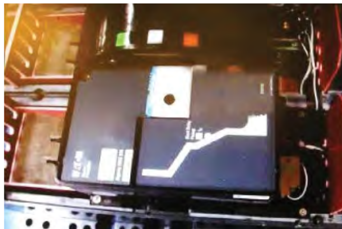
Figure 2. Trip Unit to Be Removed.
