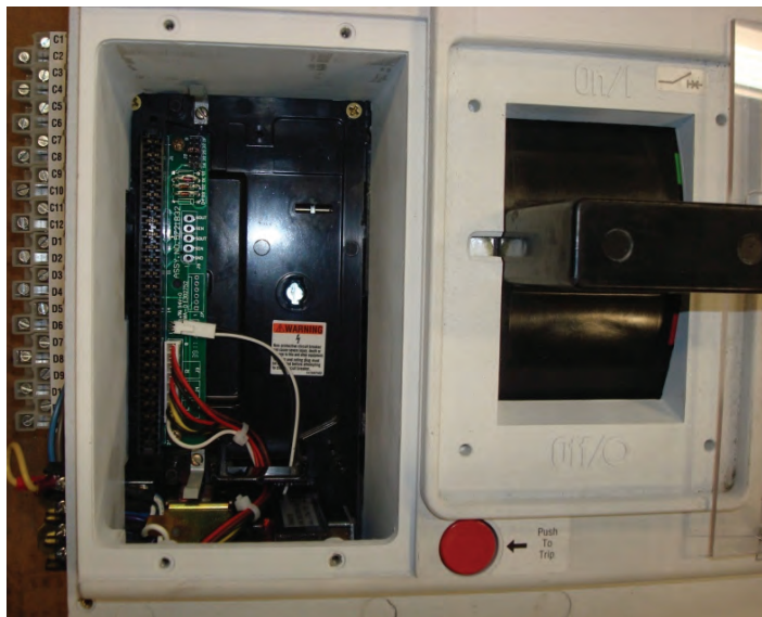
Figure 6B. Trip Unit Removed and Type "C" Edge Connector Revealed.
