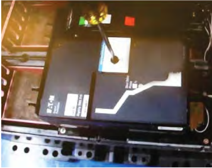
Figure 3. Unlocking the Rating Plug.
