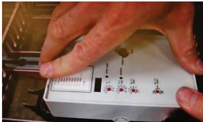
Figure 15. Installing the RG 310+ Trip Unit.
