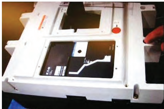
Figure 1. Trip Unit Clear Cover Removed.
