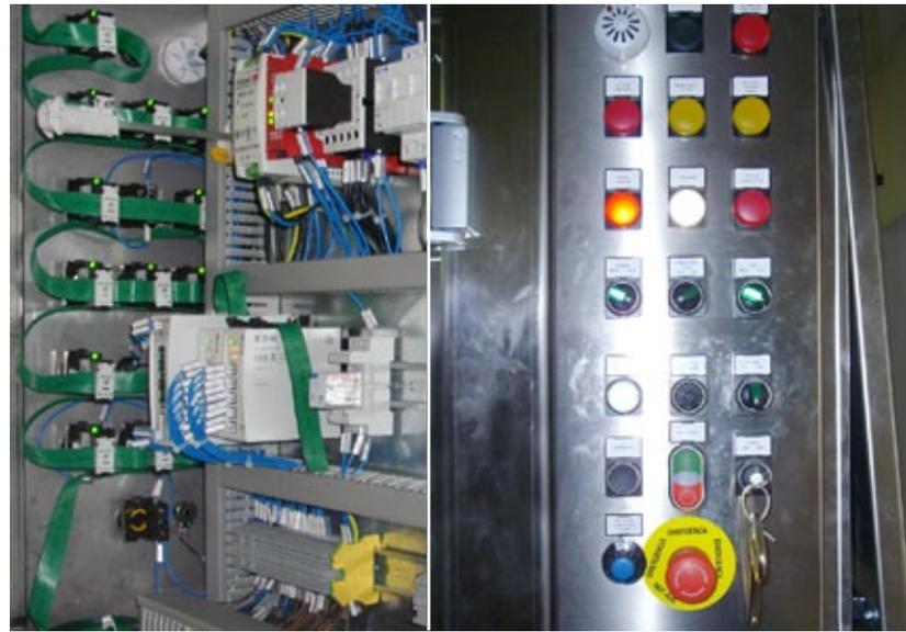
EFC chose a solution including PKZ motor protective circuit breakers, DILM contactors, Easy806 control relay and SmartWire-DT
