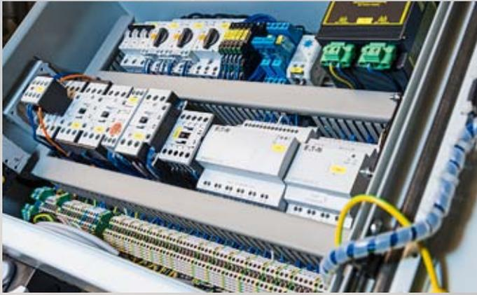
In the switch cabinet, the easy821 control relay, PKZ motor protective-circuit-breakers and DIL contactors ensure safe, reliable operation.
