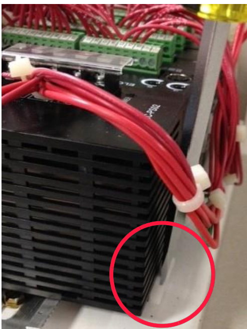
Figure 5. Unlock the Din-Rail for the Power Supply.
