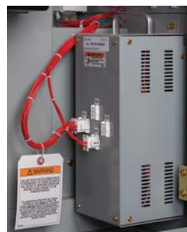
Multi-tap control power transformer
