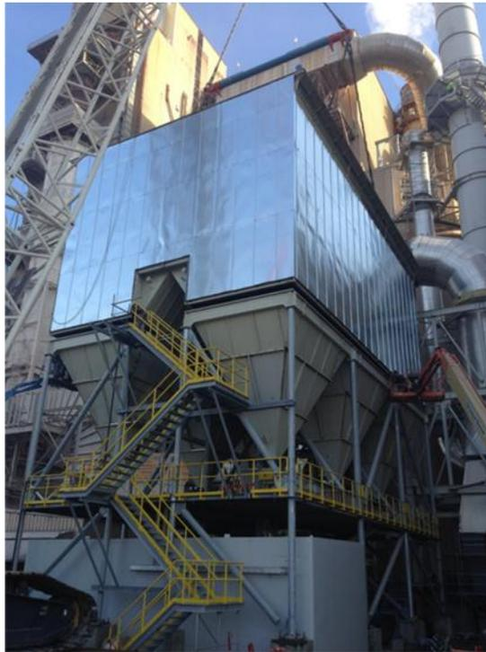
Fig. 4 New baghouse structure installed at the existing cement plant
