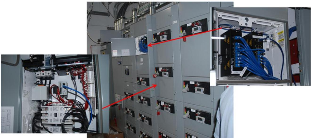
Fig. 6 Installed motor control center showing a starter unit at right and home-run connection to Ethernet switches at left
