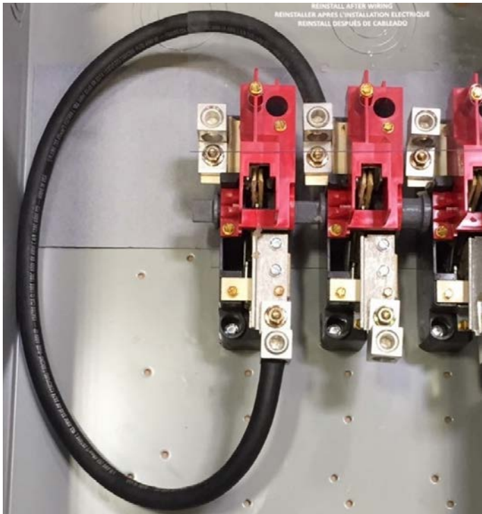
Figure 2. Sample two-pole 600 V heavy-duty safety switch
