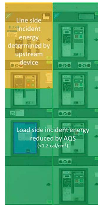
**Figure 2. Standard application incident energy**
