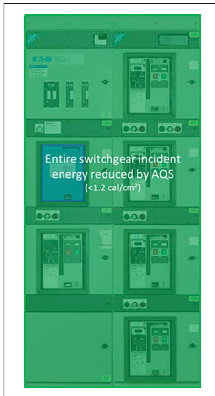
Figure 20.5-4. Substation Application Incident Energy
