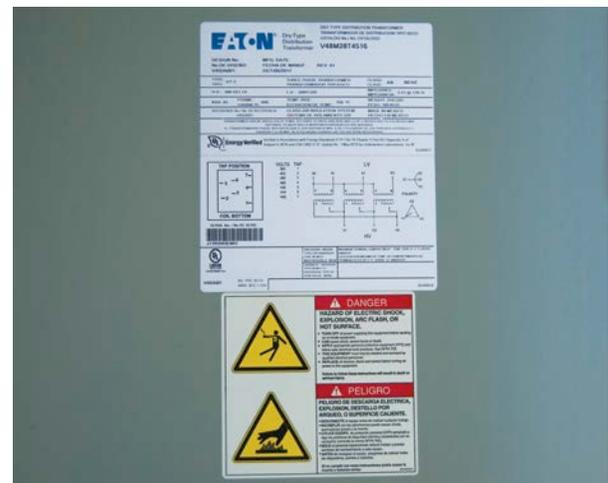
Low-voltage dry-type transformers typical nameplate information
