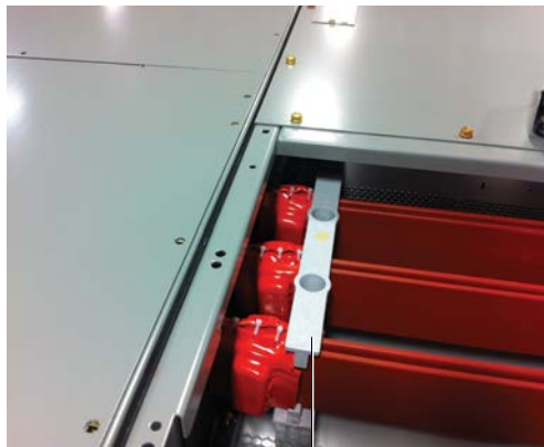
Main Bus Splice Between Unit Split
