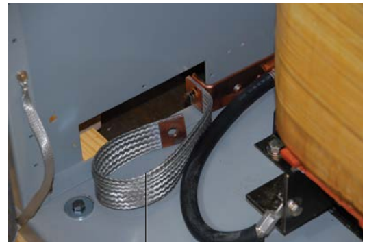
Shunt Pre-Connected to One End of Split for Shipping
