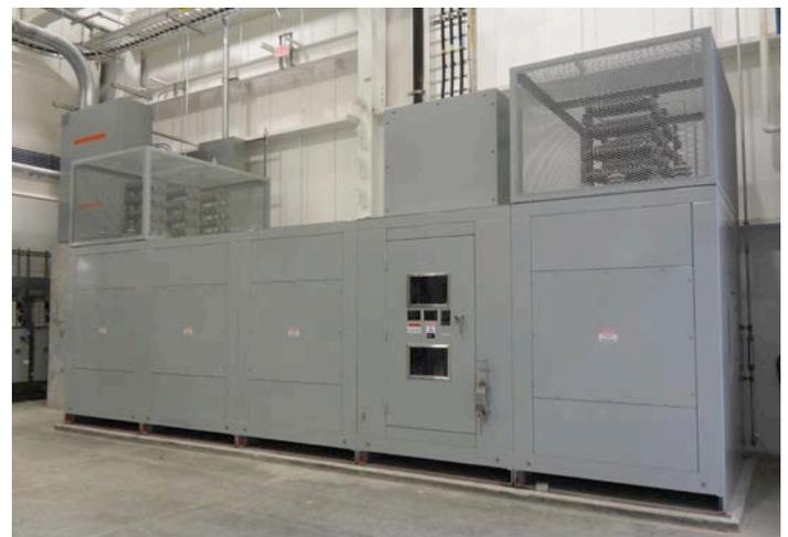
Used as a multiple-step, second-order harmonic filter bank in a large wind-turbine drivetrain facility
