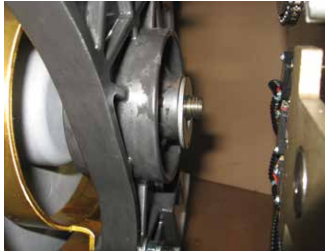
Figure 19. Installing main shaft.
