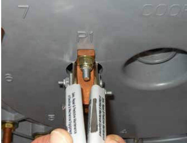
Figure 17. Installing ring into P1 contact.
