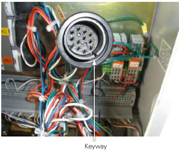
Figure 6. Male pigtail harness connector.
