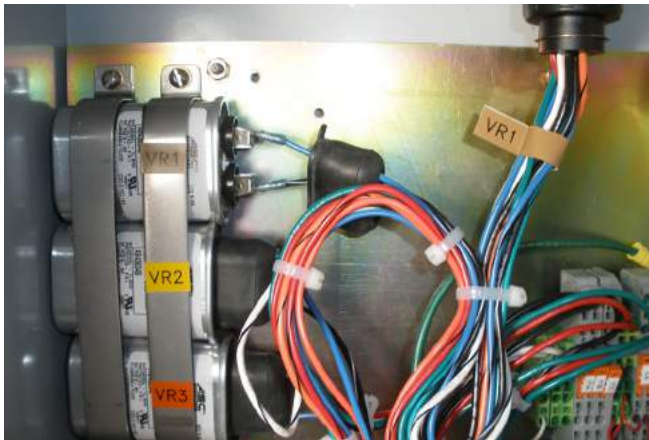
Figure 13. Alternate motor capacitor mounting provisions.
