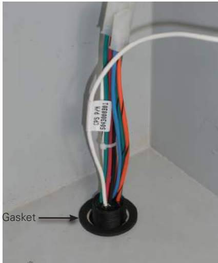
Figure 32. Pigtail internal gasket installation.
