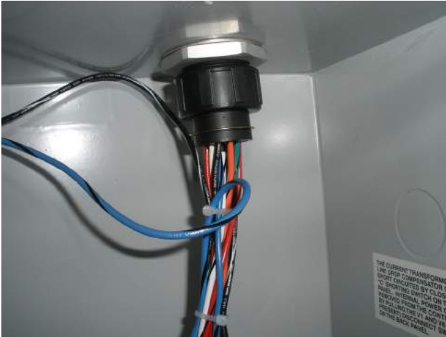
Figure 20. Installed pigtail connector on control cable.
