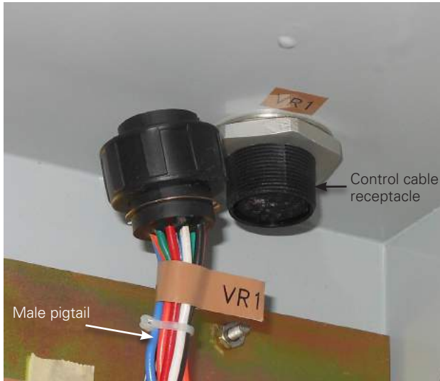
Figure 5. Coordination of control cable with pigtail harness.
