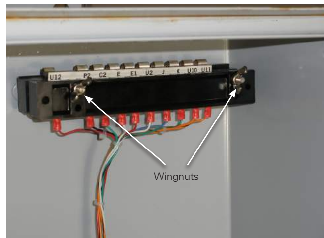
Figure 34. Wing nut installation.
