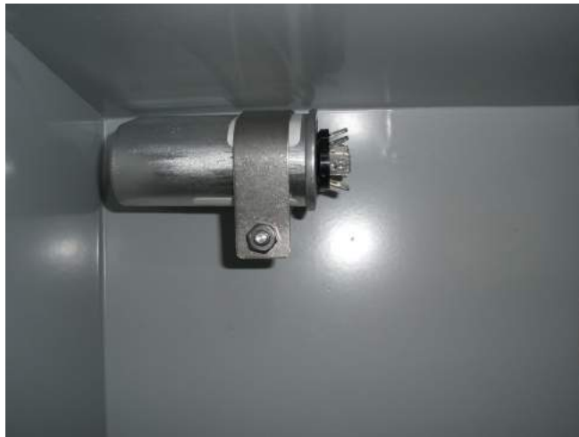
Figure 24. Motor capacitor mounting provision.
