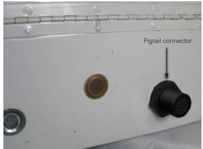
Figure 31. Installation of the pigtail into the bottom of the control box.
