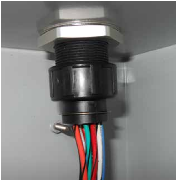
Figure 11. Connecting the control box pigtail to the universal junction box.
