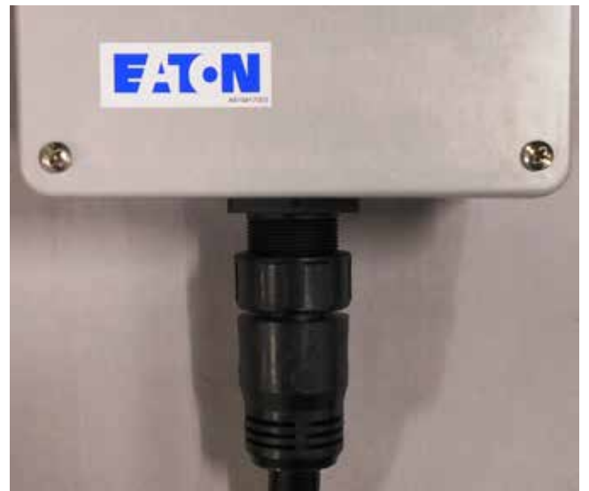
Figure 10. Connecting a quick connect control cable to the universal junction box.
