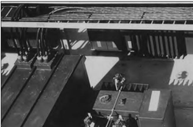
**Cables Exiting 480 Volt Outdoor Switchgear and Entering Cable Tray System** (Cable fittings with clamping glands are required to prevent moisture flow into equipment due to the cable's overhead entry into the switchgear enclosure).
