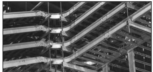
Most cable trays are utilized as continuous beams with distributed and concentrated loads. Cable trays can be subjected to static loads like cable loads and dynamic loads such as wind, snow, ice, and even earthquakes. The total normal and abnormal loading for the cable tray is determined by adding all the applicable component
