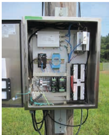
Figure 2: An Intelligent Distribution Automation Node deployed in the field
