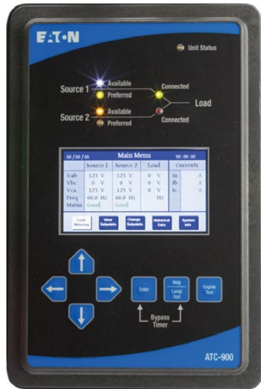
Figure 10. Automatic transfer control interface
