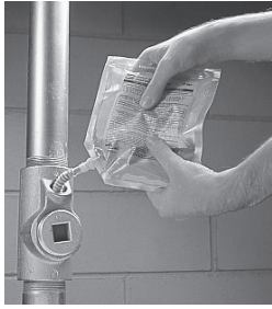
CHICO A-P INTRAPAK® premeasured sealing compound and water in plastic mixing pouch
