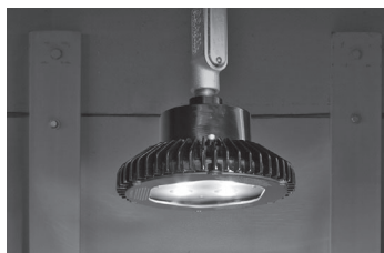
VAPORGARD™ luminaires in oil refinery
