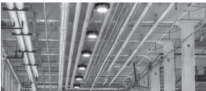
Class II luminaires allow lights to be placed where they are needed most, without fear of causing a fire from sparks or overheating.
